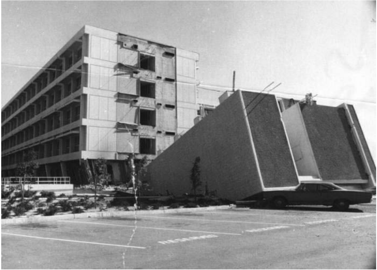
Damage to Olive View Hospital 1971 Earthquake
